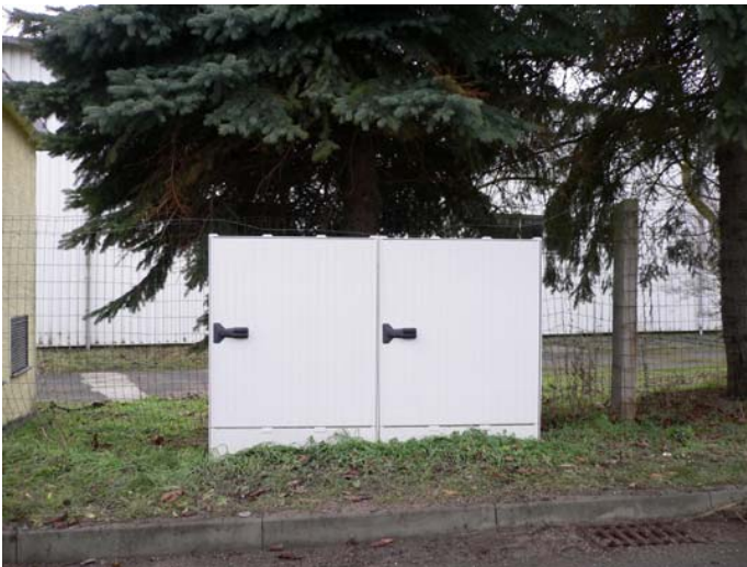
GSAB cable distribution cabinet made with SMC-technology
